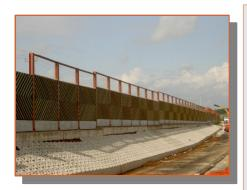
Several benefits are supposed: in addition to a high absorption capacity and to a consequent reduced acoustic reflection demonstrated by appropriate tests, the prototype can also perfectly integrates under an aesthetic point of view in the environment; therefore, it can be suitable for installation in places which require a low visual impact, like landscape or residential areas.
