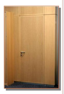
The combined use of wood and rubber with the purpose of sound absorption also finds application in indoor environments through the realization of panels applicable in walls and ceilings or suitable for the manufacture of furnishings.
